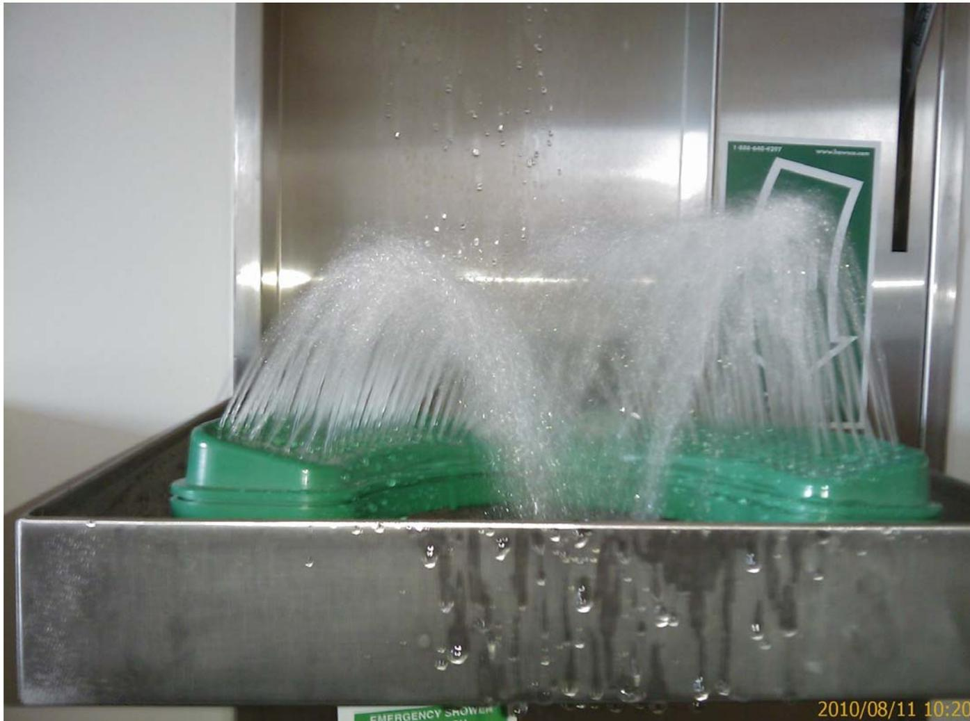
This eyewash is low flow. Note the difference in flow height vs. the pervious slide based on the sticker in the background.
