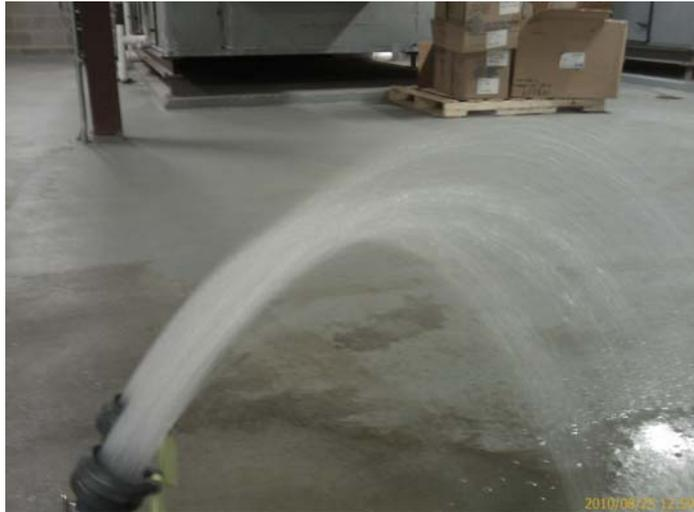
Example of good flow from a dredge hose type of safety eyewash. Note that with this type the water streams don't cross. With handle pointed strait up the streams should be about a foot long from nozzle to apex.
