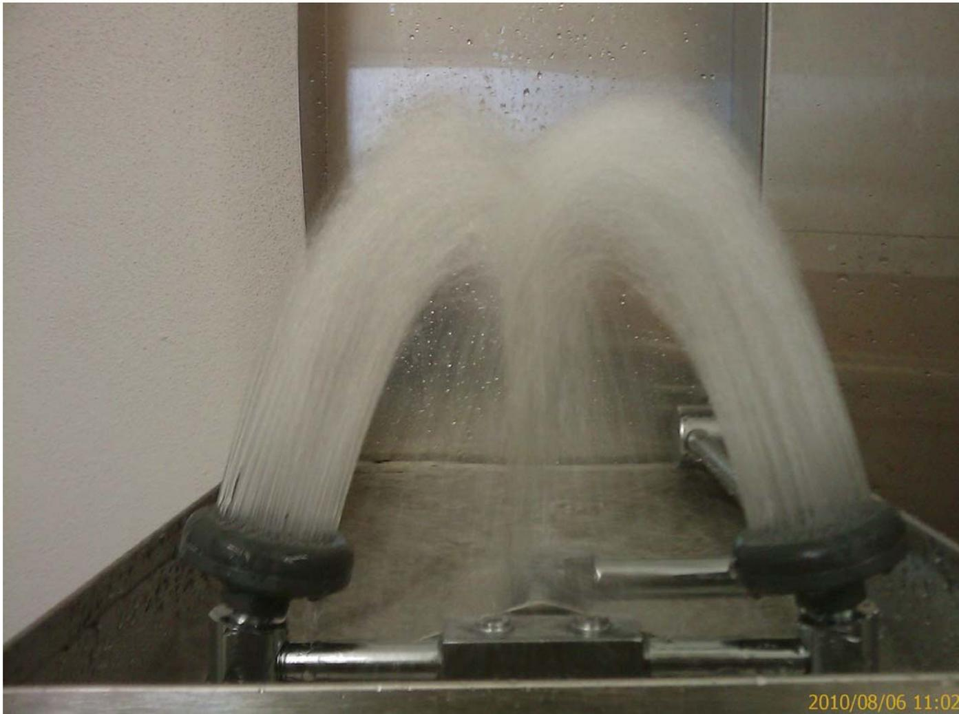
This is an ideal example of this kind of flow type. The flows are equal and cross near their apex and at the center of the eyewash mount.
