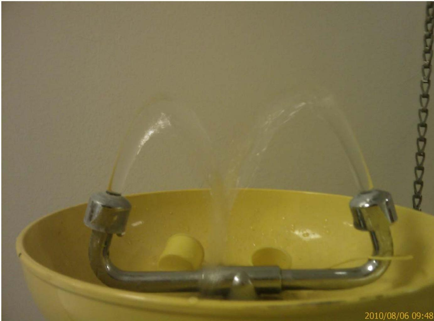
This eyewash is also deficient. The flows are low don't intersect one another. The flow while low could work in an emergency.
